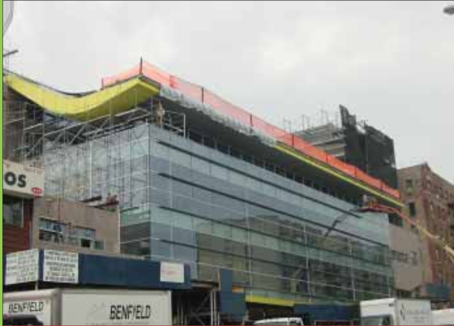
Bronx Borough Center Library - 2 Months To Completion
